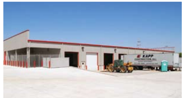
The loading area of DeLille Oxygen's new facility.
