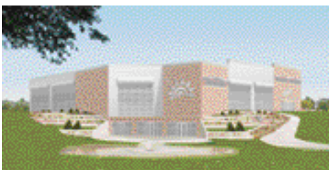
Currently under construction, West Ridge Community Church in Elgin, Ill. features a contemporary design.
